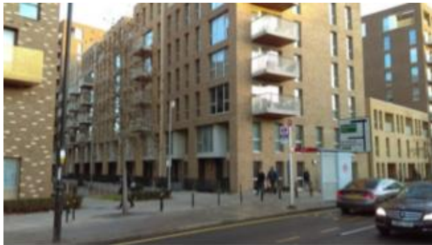
Northern footway opposite Marner Primary School, showing good quality pedestrian infrastructure
