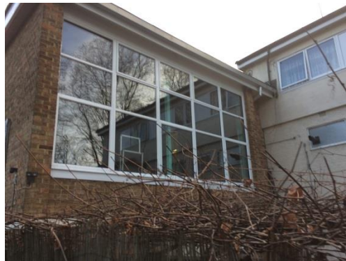
School hall with plant room flue and site manager's flat to the right. These rooms face onto the staff car park
