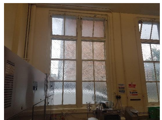
Internal – Single glazed windows
