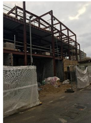
Construction site opposite Year 5/6 playground
