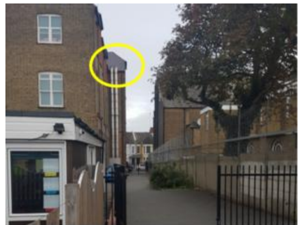
Flues from boiler terminate at eaves level
