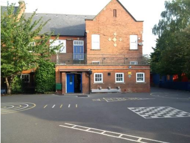
Single storey kitchen extension
