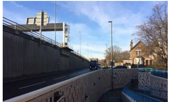
Pedestrian subway under the North Circular (and Southend Avenue)
