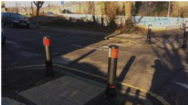
Informal crossing on approach to pedestrian subway (with 'stop look listen')
