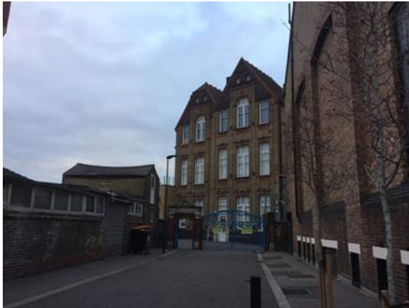
High St North school entrance approach
