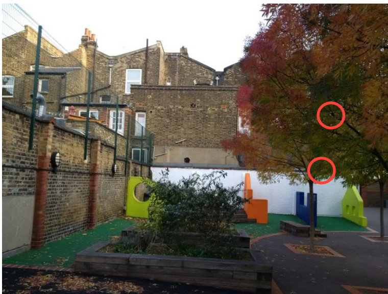
Gas boiler flue and dry cleaner extract positioned into playground
