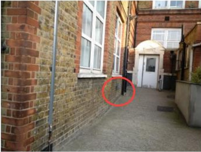
Gas heater flue at rear pupil entrance and below opening window
